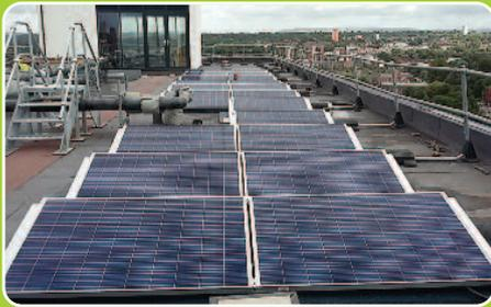
"The sheets worked very well. There are 29 panels on the roof . . . with sheets supporting a total of 4.5 tonnes of ballast blocks within the frames. We will certainly use these again."
